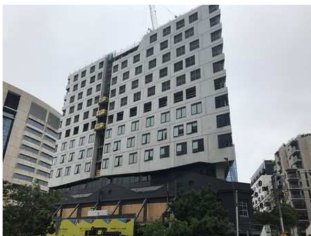
Construction of University Square, Melbourne
