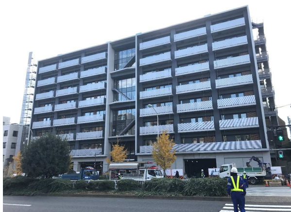
Construction of Hakusan House, Tokyo
