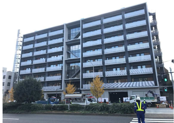
Construction of Hakusan House, Tokyo
