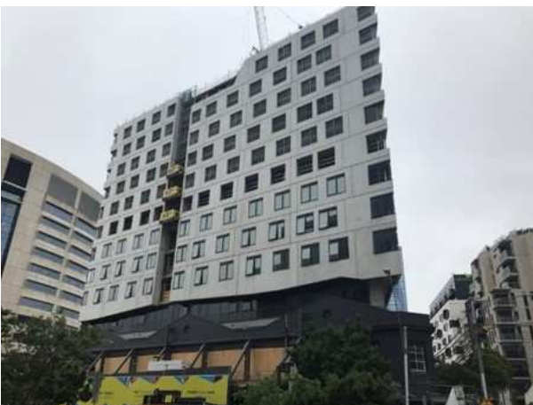
Construction of University Square, Melbourne
