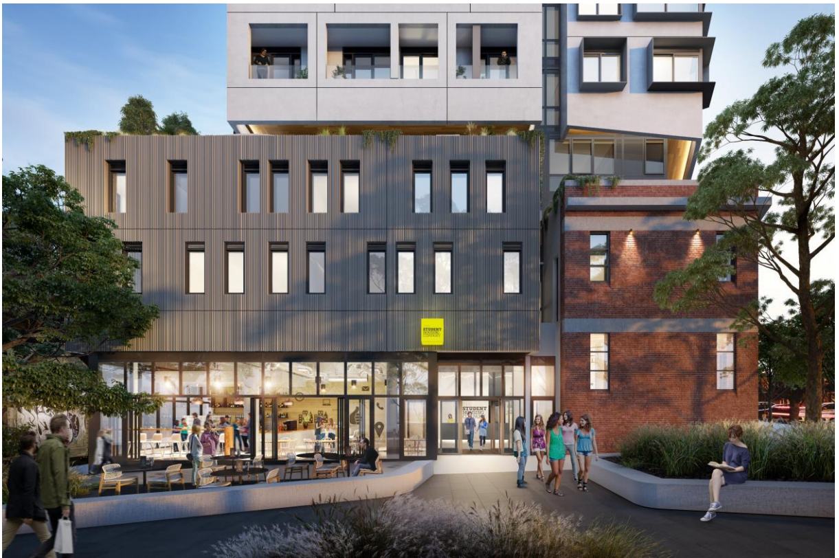
CGI of the main entrance into University Square, Melbourne – opening July 2018
