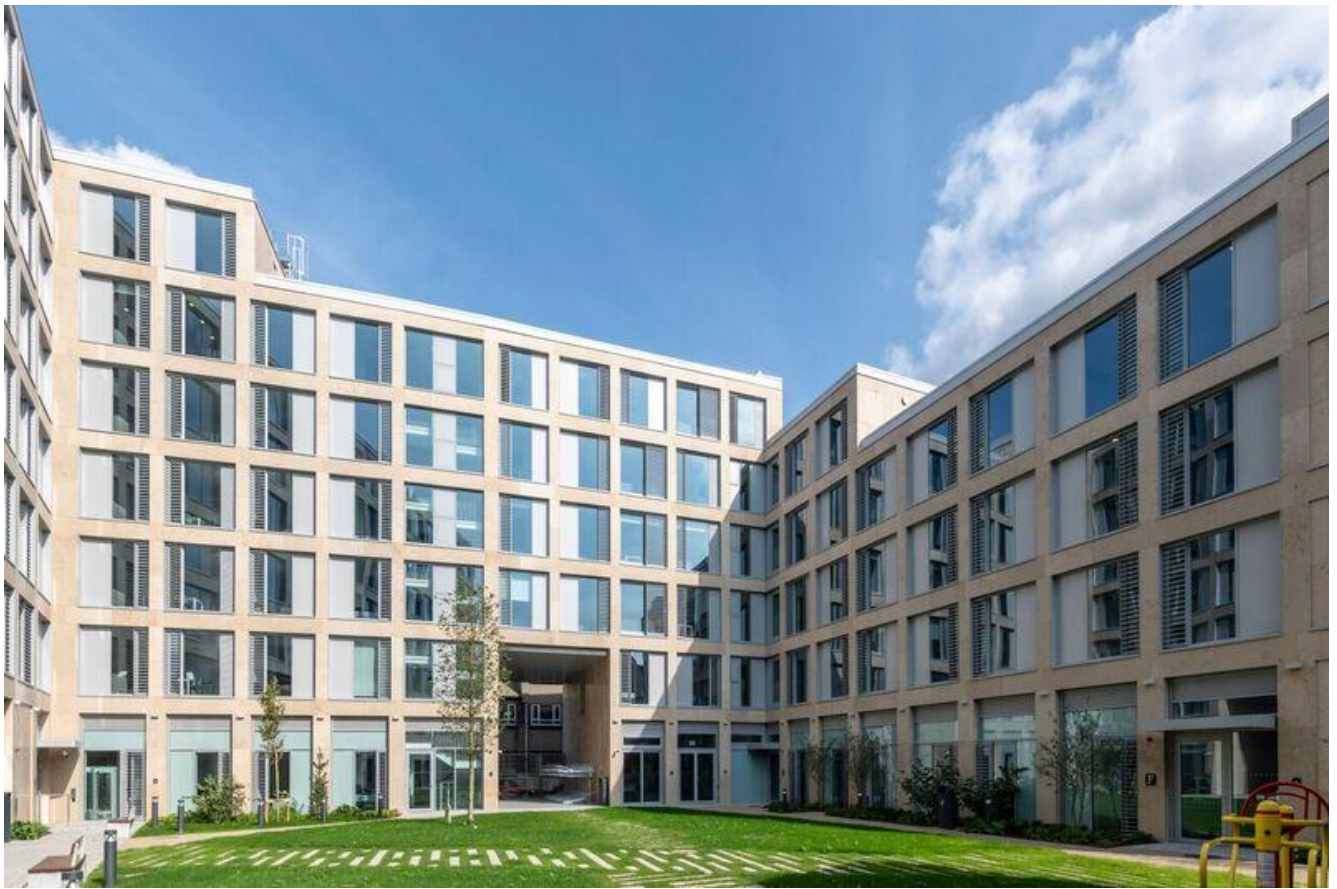
External façade of The Tannery in Dublin, Ireland
