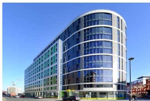
External façade of Ablett House, Liverpool
