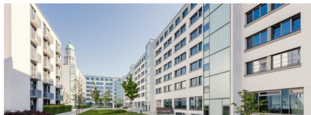
External façade of Frankfurter Tor, Berlin
